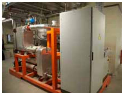
Meran (Bozen) - Heat recovery from cooling jackets and exhausts of gasifiers and syngas-fueled engines
