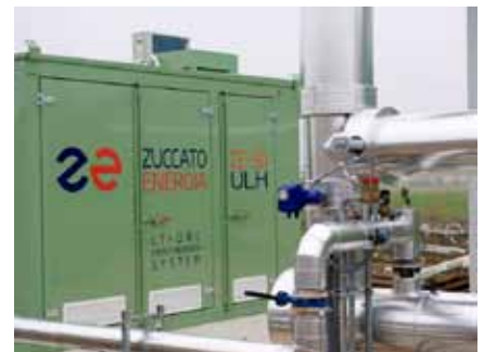
Borgoforte (Mantua) - Heat recovery from cooling jackets and exhausts of biogas-fueled engines
