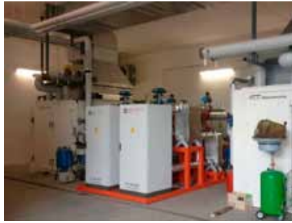
Renon (Bozen) - Heat recovery from cooling jackets and exhausts of vegetable oil-fueled engines
