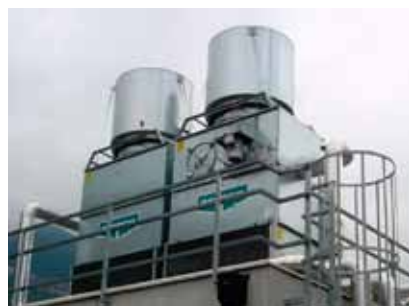
Optional silencing system for residential area applications
