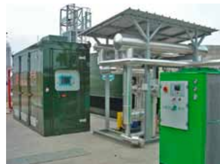
Portogruaro (Venice) - Heat recovery from cooling jackets and exhaust gases of biogas-fueled engines
