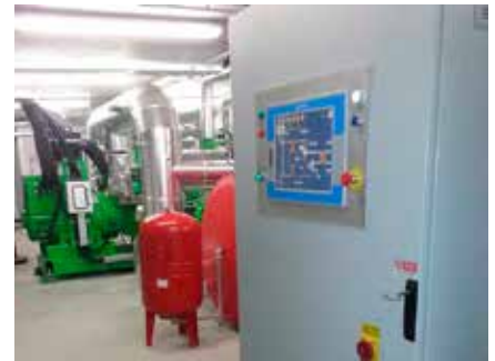
Morgex (Aosta) - Heat recovery from cooling jackets and exhausts of vegetable oil-fueled engines
